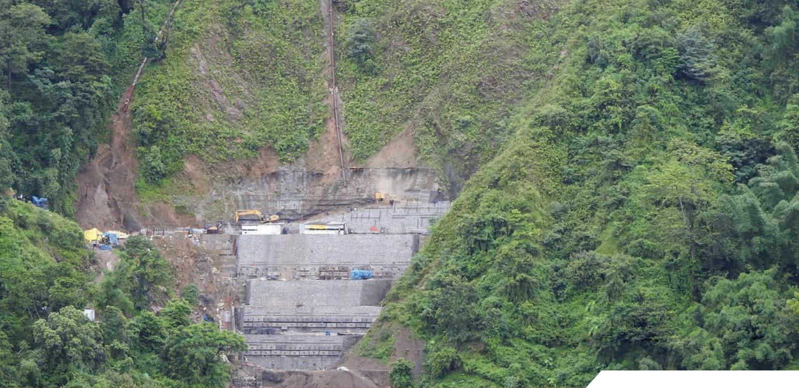
presence of natural aquifer. Therefore, while drilling the holes for nail, significant water flow was encountered. Long semi-perforated pipes were installed within the slope to cater to this challenge.
