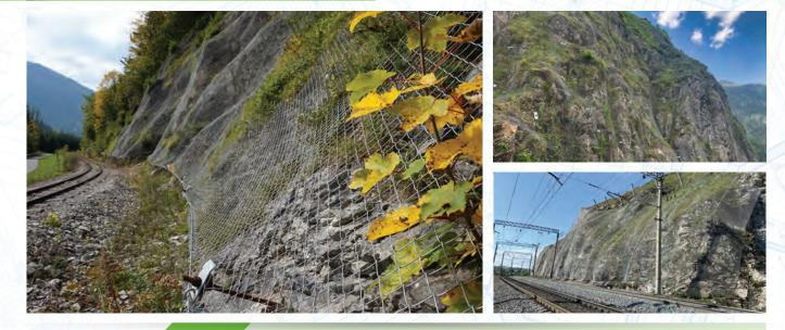
Terre Armée offers engineered solutions for **Slope Retention** to retain the masses in situ and prevent erosion and shallow landslides. This systems is designed on a site to-site basis. Depending on the site characteristics and strength requirements, a large variety of net and netting products are available. Re-stabilization of the slope using mesh and natural vegetation is highly encouraged. Furthermore, netting can accommodate pre-existing vegetation such as tree trunks with minimal effort.
