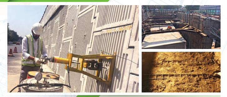
**ReMain®** is a specific selection of techniques used to maintain, strengthen and upgrade Reinforced Earth® structures. **ReMain®** is used for restoration and strengthening of existing structures (typically retaining structures, bridge abutments, wing walls and return walls). The durability, service life and performance of the affected structure can be significantly improved.
