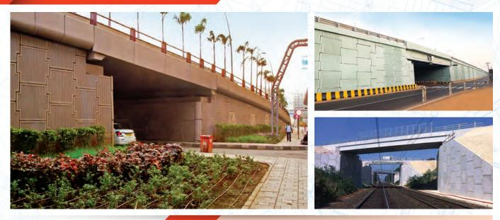
**TechAbutment**<sup>®</sup> is an alternative solution for RCC / piled abutments. A highly engineered technique, it has been adopted throughout the world successfully for over 40 years. It is a Reinforced Earth<sup>®</sup> structure designed to support bridge load as an alternative to conventional RCC abutments. This is used for bridges, underpasses, flyovers, ROBs and RUBs.
