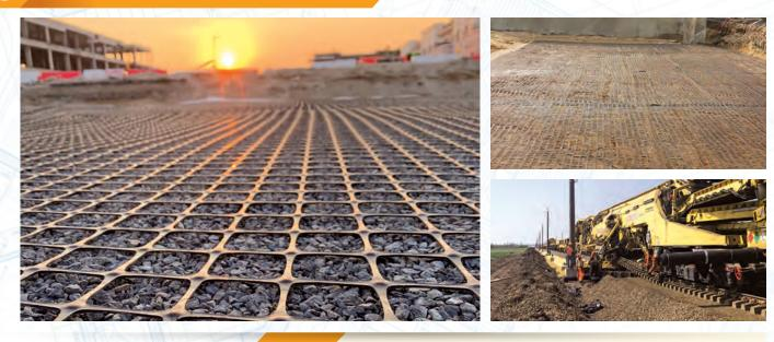
ArmaGrid<sup>™</sup> is a uniaxial or biaxial geogrid made from either polyester or polypropylene or HDPE. It is used as soil reinforcement in various applicatons such as foundation improvement, trackbed stabilization, basal reinforcement etc. Terre Armée India uses in-house design capacity to select the type and strength of material based on the actual site condition.
