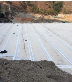
**TerraDrain**<sup>®</sup> is modular light weight, high strength and high impact cellular drain board wrapped with a custom designed geotextile and used for subsurface drainage. The drainage board and the non-woven geotextile used in **TerraDrain**<sup>®</sup> are manufactured from polypropylene. The open surface design and high internal void volume enables the rapid capture and transport of high amount of water.
