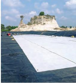
**TerraLine**<sup>®</sup> Geosynthetic Clay Liners (GCL) are factory made hydraulic barriers consisting of very low-permeability bentonite powder supported by geotextiles and/or geomembranes. The engineering function of a **TerraLine**<sup>®</sup> - GCL is containment as a hydraulic barrier to water, leachate or other liquids and sometimes gases.
