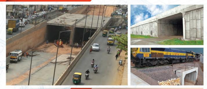
**TechBox**<sup>®</sup> is a state-of-the-art precast 'box' structure, typically a oneor three-segment system suitable for cut 'n' cover buried structures. The precast segments are brought to the installation site, when the site is ready for construction. It allows rapid on-site regulated installation. The soil cover required in **TechBox**<sup>®</sup> structures is lower than for arch structures.
