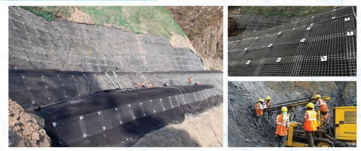
**TerraNail**<sup>®</sup> is an in-situ method of reinforcing existing soil/rock mass by installing solid or hollow fully threaded hot-dip galvanized high tensile geotechnical steel bars encased in grout. **TerraNail**<sup>®</sup> is typically use to stabilize existing slopes or excavations. It is also a reliable solution for landslide rehabilitation and active rockfall protection.
