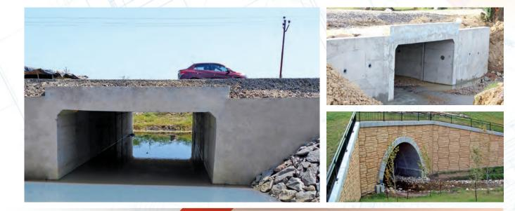
**TechCulvert**<sup>®</sup> is small to medium sized single unit Precast 'Box' or two-pin Precast 'Arch' for hydraulic culverts and utility covers (like gas pipelines). **TechCulvert**<sup>®</sup> provides several benefits to project owners, like assured quality, savings in indirect cost, rapid construction and early traffic commissioning.
