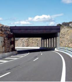
Rockfall is an inherent hazard of mountainous terrains, which jeopardizes life, property and threatens the smooth operations of traffic lines. **TechShelter®** is a perfect custom-designed solution of pre-cast arch box (TechBox® and TechSpan®) for sheds and shelters to suite these site conditions. This is one of the most reliable, cost-effective system for cut 'n' cover structure.
