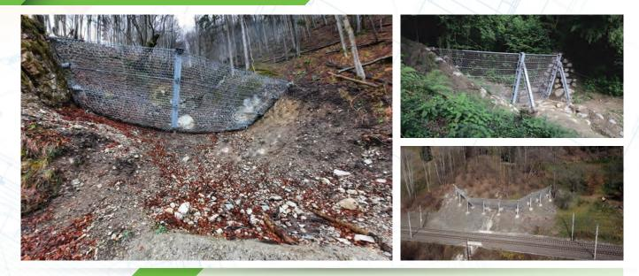
Terre Armée offers engineered solutions to protect infrastructure, and assets from debris flows and debris floods. The threat of climate change raising the global temperatures, potentially causes a change in weather patterns, thawing of permafrost areas, increasing wildfires, debris flows, and shallow landslide activity. The use of flexible-net barriers can be an efficient alternative to the other traditional and costly mitigation measures such as dams and other rigid barriers.
