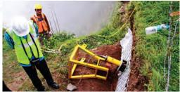
TerraAnchor™ technology is an active soil reinforcement system used for permanent as well as temporary stabilization of existing slopes / structures by using high tensile steel as soil reinforcement (galvanized bars for permanent and strands for temporary). It is a driven and stressed soil anchoring system used with suitable facing.
