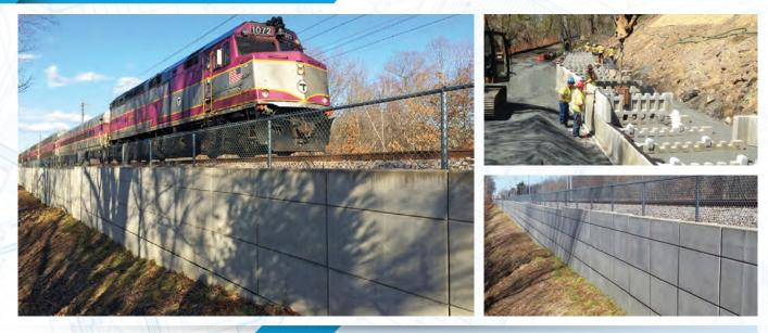
The **T-Wall**<sup>®</sup> system is a precast modular gravity type reinforced concrete retaining wall system. It is most suited for railway load supporting structures and construction of submerged retaining structures. The **T-Wall**<sup>®</sup> system decreases in stem length course by course – reducing materials, excavation and backfill as compared to other wall systems.
