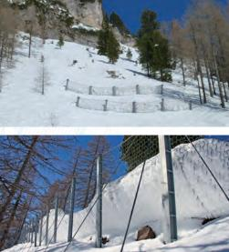
Avalanche Barrier systems are designed on a site-to-site basis to protect infrastructure, utilities, buildings, reforestation, and lives from avalanches. Snow nets, snow rakes and steel snow bridges are installed in the initiation zones to prevent avalanches from forming. Static defense structures, snow catchment fences/ barriers are used which effectively reduces the run-out length of an avalanche.
