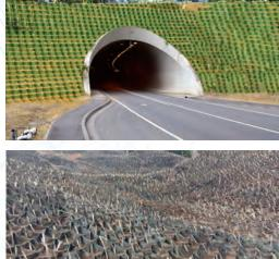
ArmaWeb® is a 3-dimensional soil stabilization and erosion protection system. It is made of High Density Polyethylene (HDPE) and welded at junctions to form cellular confinement systems.
