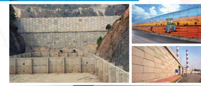
**Reinforced Earth**<sup>®</sup> structures combine engineered backfill with steel or synthetic tensile reinforcement and a modular concrete facing system. This ideal combination creates a durable and resilient earth retention structure. With **Reinforced Earth**<sup>®</sup> structures we can create several attractive architectural finishes.
