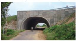
**TechSpan**<sup>®</sup> is a one of the most reliable, cost effective precast concrete arch systems available for cut 'n' cover structures. It is widely used in the construction of bridges, underpasses, conveyance and reclaim tunnels, portals, ammunition storage bunkers and rockfall sheds and shelters. Typically, 15-20 linear meters of **TechSpan**<sup>®</sup> can be installed in one work shift.
