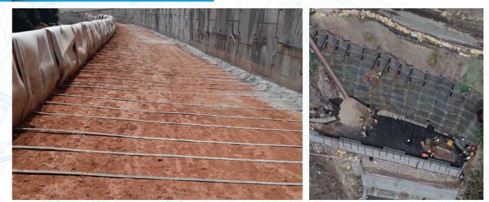
**TerraLink®** technique allows building of earth retention structures connecting existing profiles stabilized by soil nails and/or anchors. It is a useful technique for construction of benches and for road widening projects with limited available space, and activates the best optimisation between cut and fill requirements.
