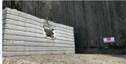
**TerraBund**<sup>®</sup> is a Terre Armée protection bund. It is a gravity structure built using soil reinforcement and flexible or semi-rigid facing systems. It is a passive protection system used typically as a geo-hazard solution against rockfalls, avalanches, debris flow and mud slides. **TerraBund**<sup>®</sup> can withstand more than 8000kJ of impact energy in the event of landslide or rockfall.
