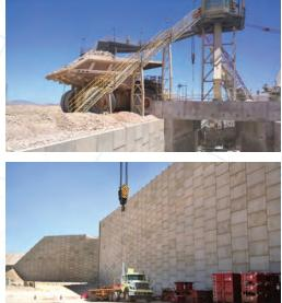
**Composite Earth**<sup>®</sup> technology adopts primary and secondary soil reinforcement systems for the design of Reinforced Earth<sup>®</sup> retaining walls. It aims to control the lateral deformation of the facing during construction and operation, including during seismic events. This is an effective way to design and construct tall and critical structures.
