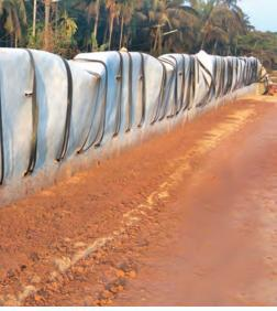
**TerraFlow**<sup>®</sup> Geocomposite consists of bi-planar High-Density Polyethylene (HDPE) geonet having non-woven polypropylene (PP) geotextile heat bonded on both sides. Bi-planar geonet is designed with two HDPE strands crossing each other at a constant angle to form a diamond structure to provide better planar waterflow under high loading. Tri-planar geonet consists of three HDPE strands to improve the lateral drainage and transmissivity.
