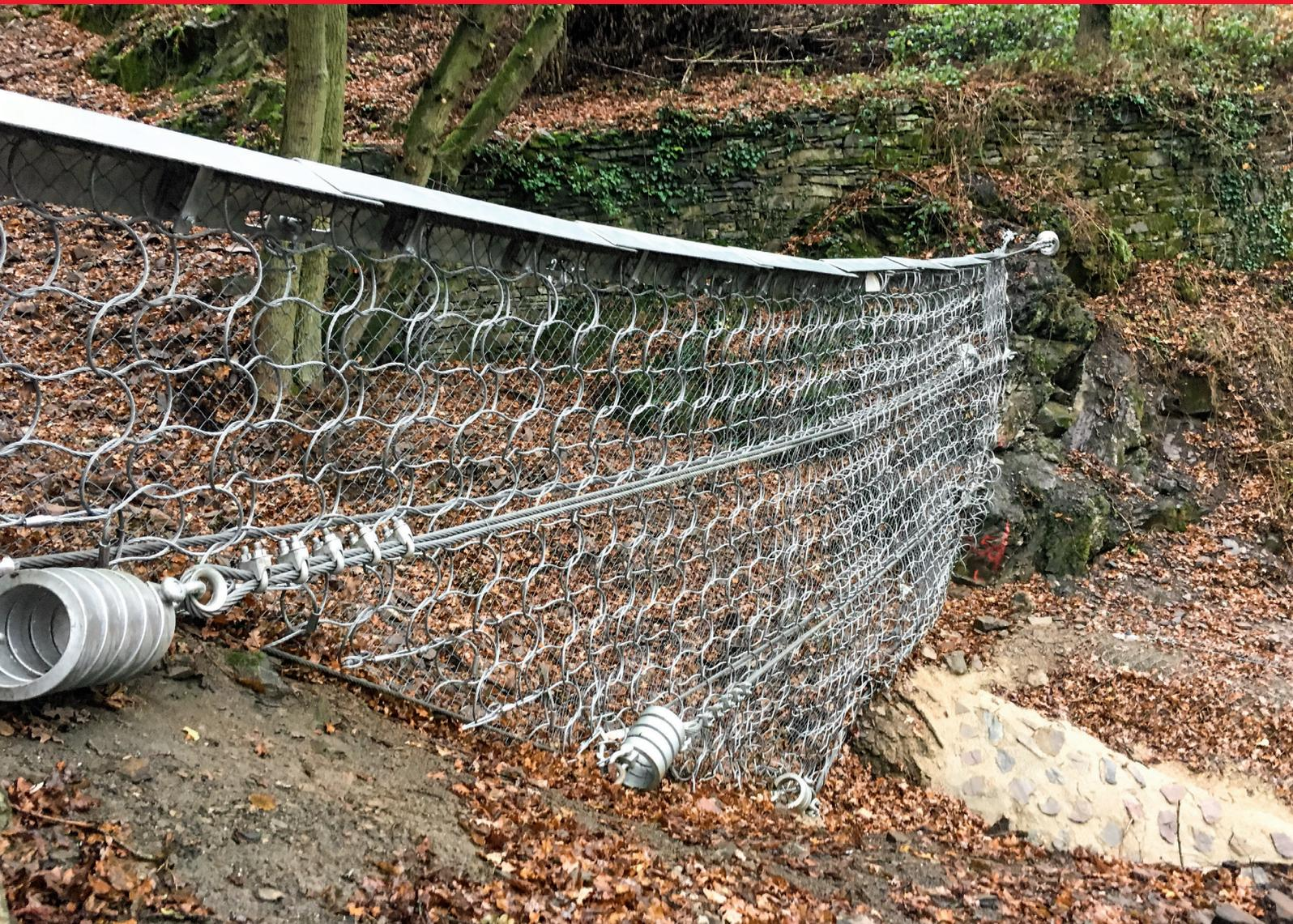
Gully nets are the simplest style of debris flow barrier. They are designed to be installed in topographically confined channels, typically up to approximately 15 m in width. The shape and gradient of the channel have a large influence on the retention capacity of the system. When in steep terrain, they are often used in cascading series to help successively remove the debris along the transportation zone of the debris flow.
