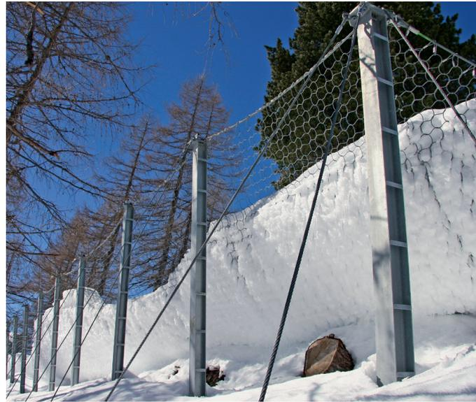
Avalanche protection systems are designed on a site-to-site basis to protect infrastructure, utilities, buildings, reforestation, and lives from avalanches. Unlike other mitigation methods such as control through triggering with explosives, these static defence structures help to prevent snow avalanches from starting in their first stage of occurrence.
