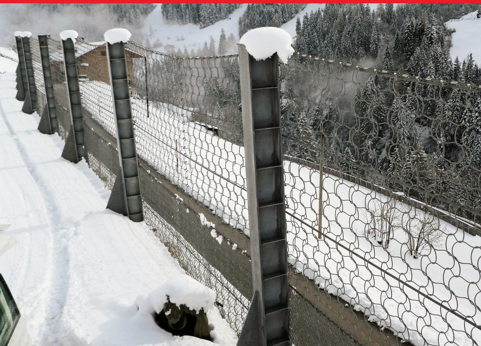
Snow catchment fences such as the SNOW-CATCHER do not prevent the initiation of avalanches but instead interact with an avalanche in the run-out or deposition zones, to slow the avalanche and bring it to a standstill. This shortens the destructive reach of avalanches.
