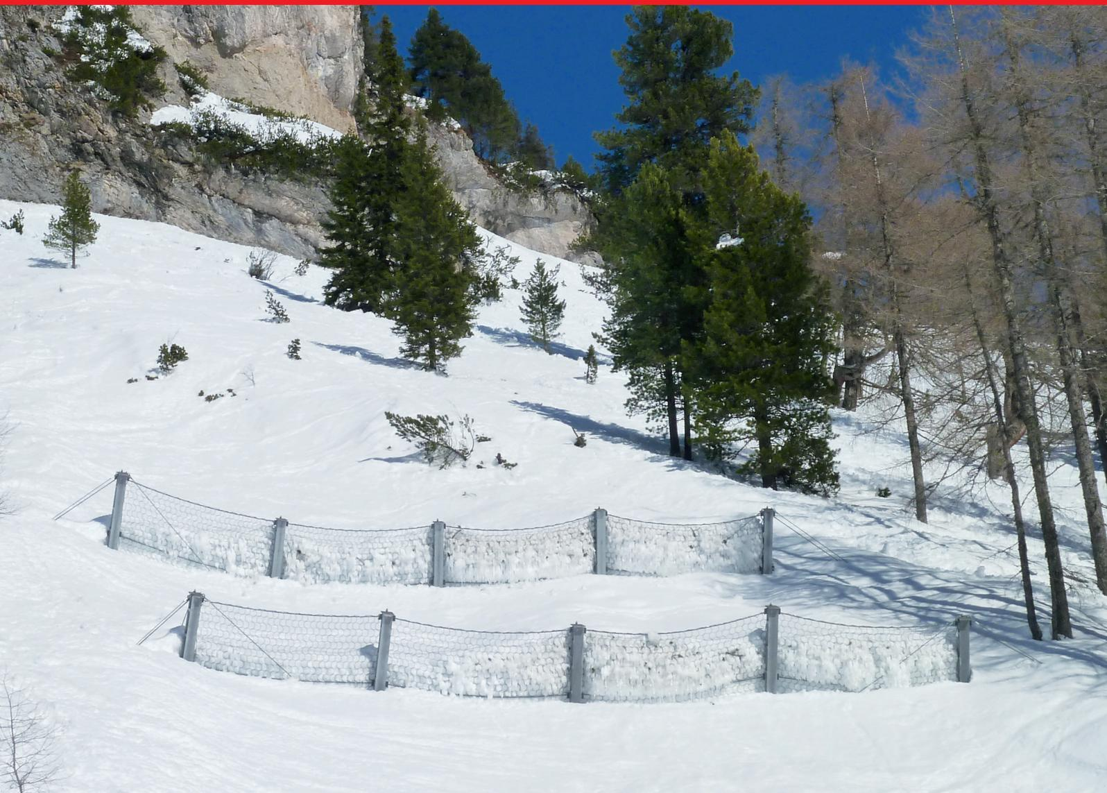
Flexible-net snow rakes are similar to snow nets as they are installed in potential initiation zones to prevent avalanches from developing.
