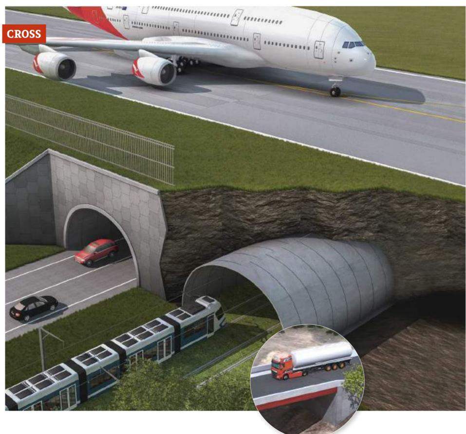
Our techniques are used to build all types of structures to meet the **CROSS**, function, such as reinforced backfill bridge abutments for overhead crossings, as well as cut-and-cover tunnels, culverts and underpasses for underground crossings.
